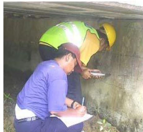
Fig 13: Rebound hammer test conducted on selected abutment
